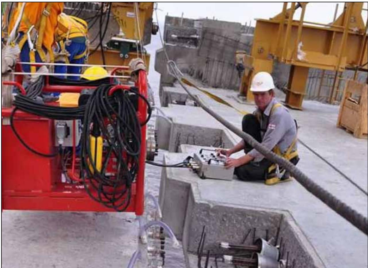
DL-M control system being used for final alignment of bridge deck sections
